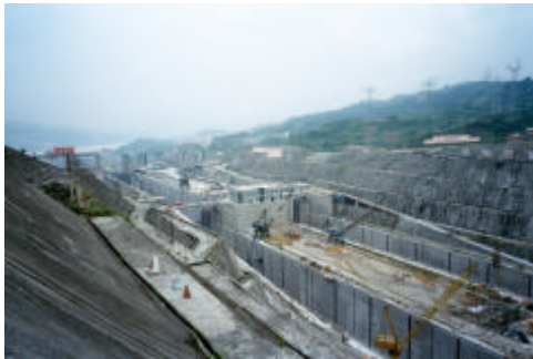
Canal construction at Three Gorges Dam, China. (Photo: W. Y. Chiau)
