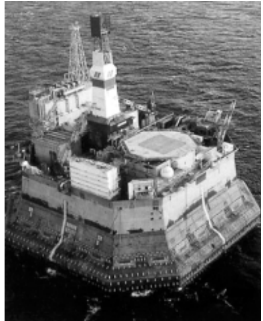
Figure 2. Molikpaq offshore platform ( http://www.offshore-technology.com )
